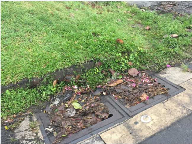
↳ Organic materials block storm drains after heavy rains, leading to drainage related flooding. Photo: Office of Planning
