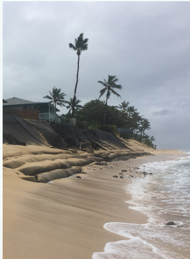
↳ Sandbags and geotextile cloth are used to protect homes from sandy shoreline erosion on O'ahu's North Shore.
