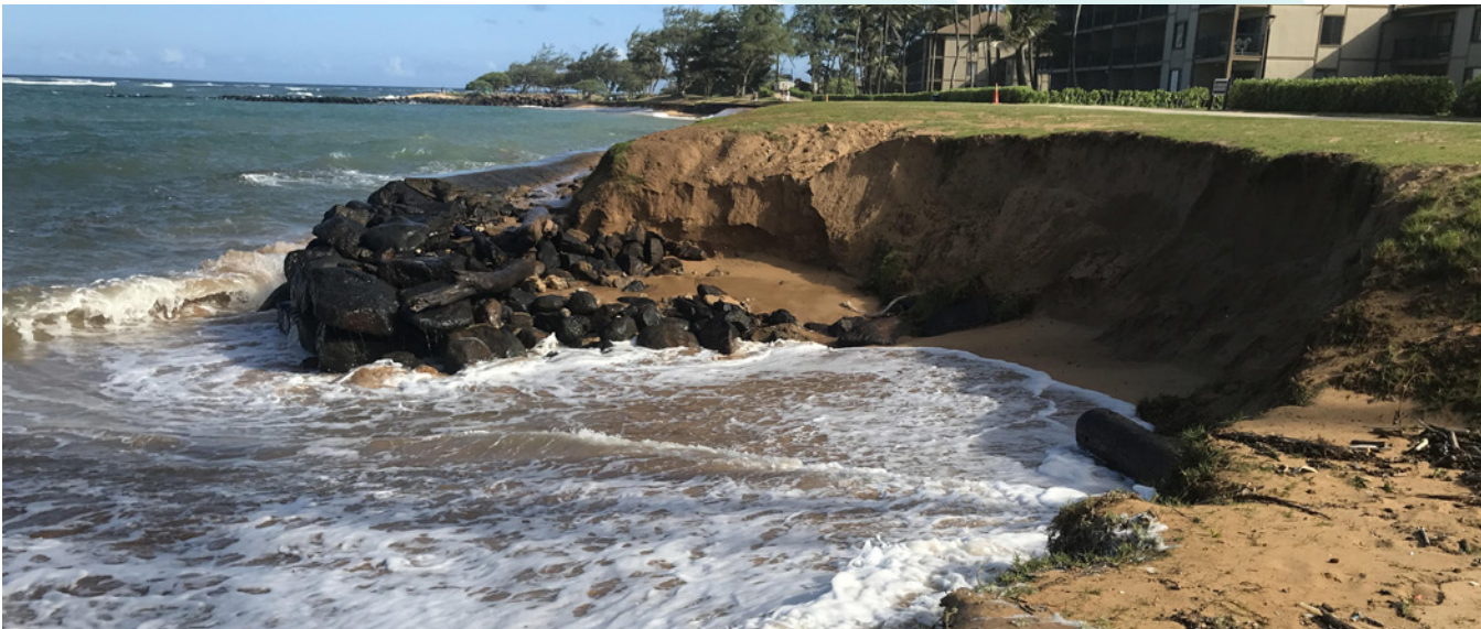
➔ A phenomenon known as 'flanking' often occurs when a shoreline structure such as a vertical sea wall is located adjacent to an unarmored sandy shoreline. Here, reflected wave energy erodes a beach area during king tide conditions at Kapa'a Beach Park, Kaua'i. Photo: Hawai'i Sea Grant King Tides Project
