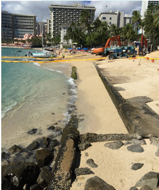
→ The construction of a 95-foot-long sandbag groin stabilizes sand on the east end of Kūhiō Beach Park in Waikiki. In the foreground, the foundation of the old Waikiki Tavern (CA. 1930's) is exposed, presenting a hazard to beachgoers. Photo: Office of Planning
