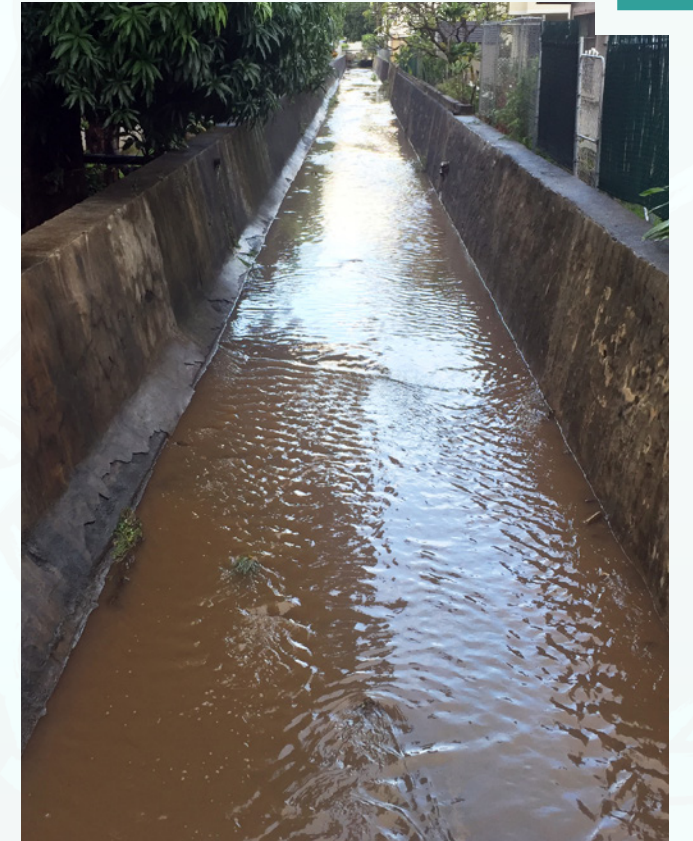
↳ Channelized streams eliminate habitat value and serve as conduits of polluted stormwater runoff. Photo: Office of Planning
